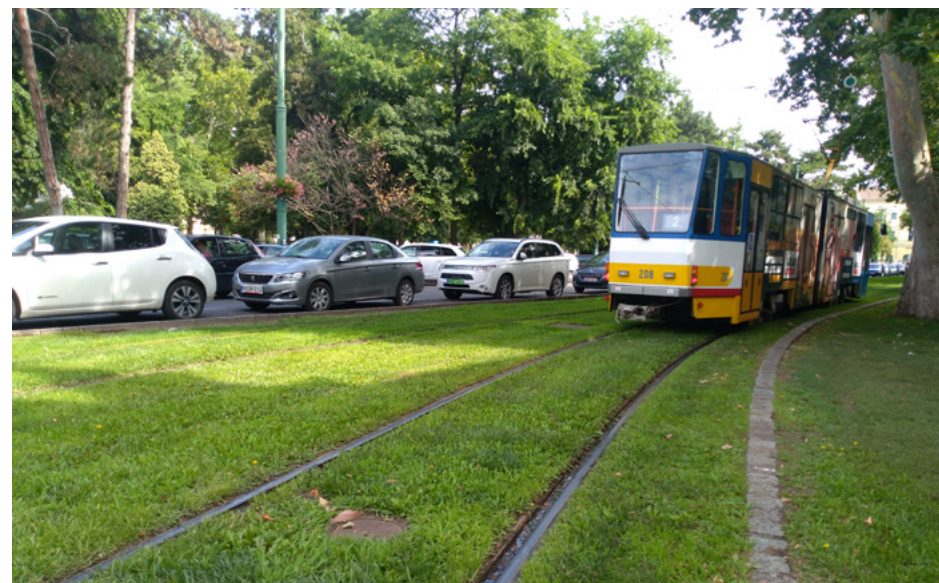
Local best practice – green infrastructure in the city of Szeged
