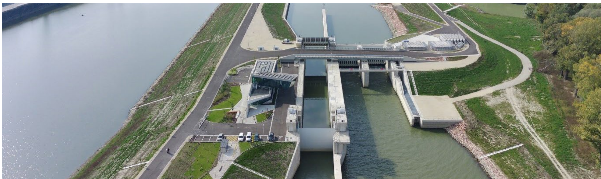
Estuary water level control structure and lock
